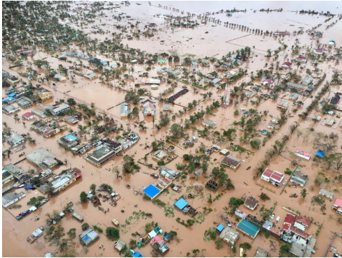
Flooding; cyclone Idai
