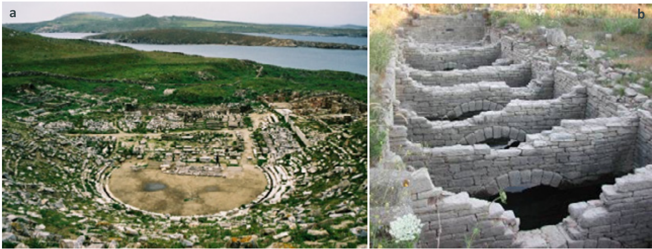
Figure 3.11 Theatre in which rainwater drainage and harvesting for reuse: (a) the theatre in Delos island and (b) the cistern used for harvesting the drainage water.
