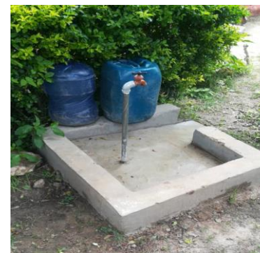
Installed standpipe with tap
