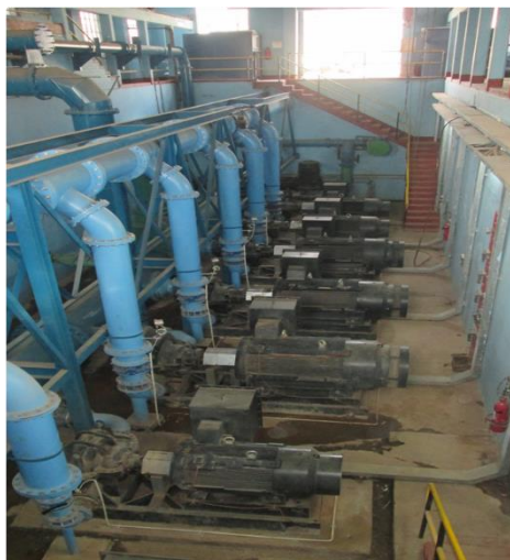
New High Lift Pumps, Motors and piping installed
