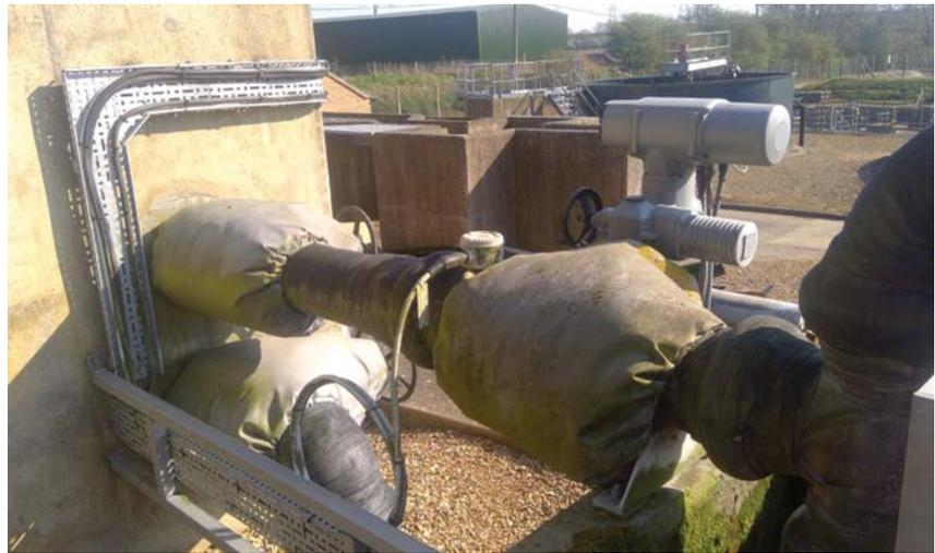
*Figure 1 Poorly installed flow to full treatment flow meter.*
