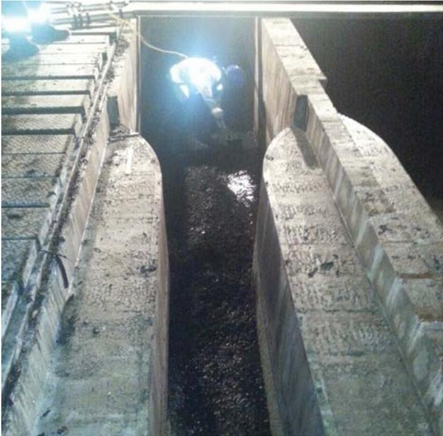
*Figure 2: A large flume influenced by poor maintenance procedures allowing grit build up.*
