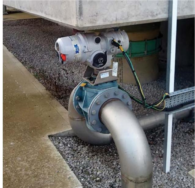
*Figure 3 – Poor installation can breed poor maintenance. This control valve, installed underneath a raised tank, is not accessible for maintenance purposes.*
