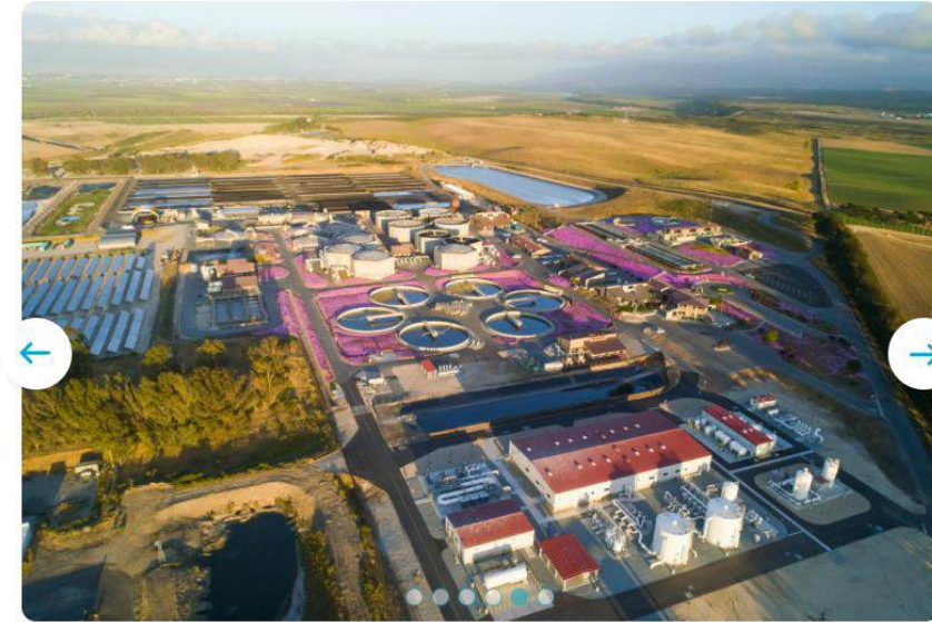
Monterey One Water, California, USA – Operating Groundwater Augmentation using 4 source waters
