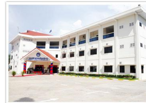
Regional Flood and Drought Management Centre in Phnom Penh, Cambodia
