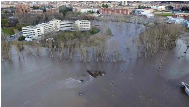
Figure 7. December 2019 flooding in the project area.
