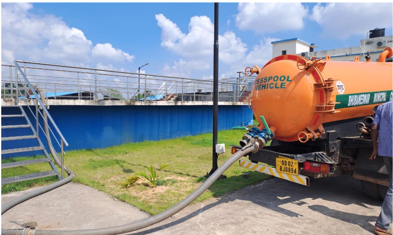
Figure 2 – Cesspool vehicle disposing sludge at the plant. Source: H&UDD.
