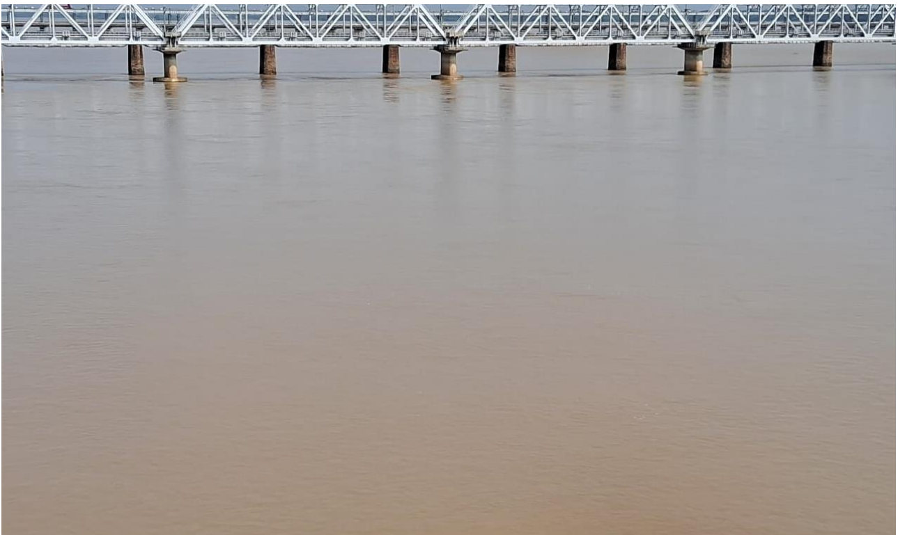
Figure 4 – Mahanadi River, Odisha. Source: H&UDD.
