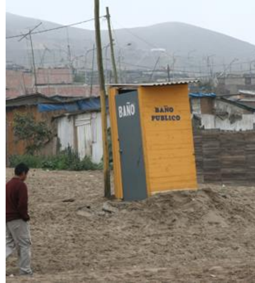
Unusable Toilets in Peru
