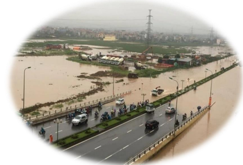
Flood in Hanoi due to heavy rain (24 th May, 2024)
